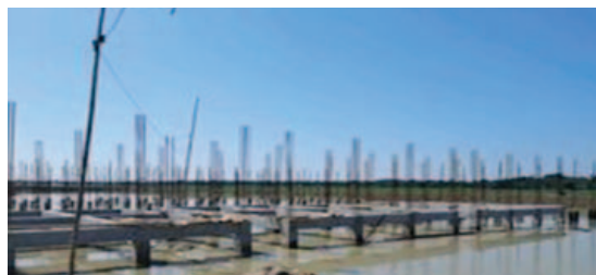
Construction of Grade Beam
